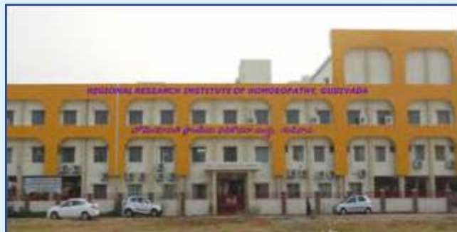
Regional Research Institute (H), Gudivada, Andhra Pradesh
